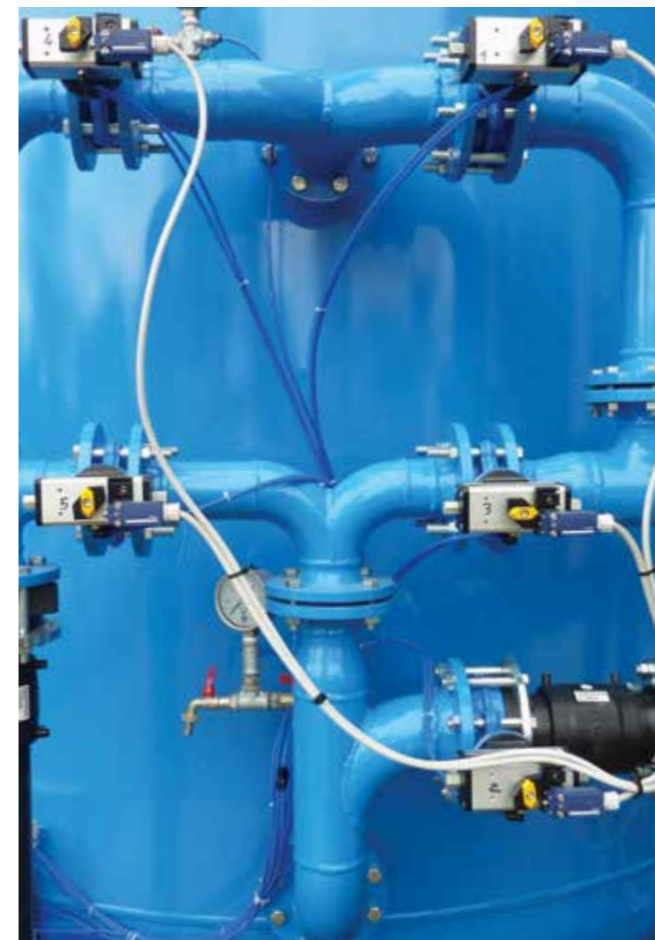
BUTTERFLY VALVES WITH PNEUMATIC ACTUATOR
