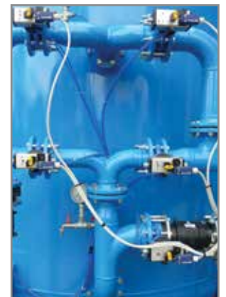
Butterfly valves w/pneumatic actuators.
